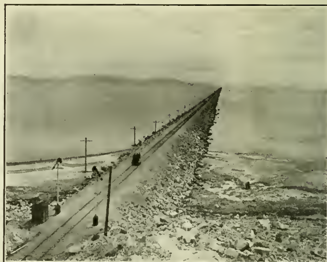
Fill Forming Easterly Portion of Great Salt Lake Cut-off
